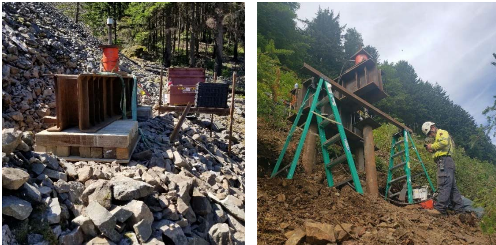
Figure 5. Preconstruction verification testing (left) and production proof testing (right)
