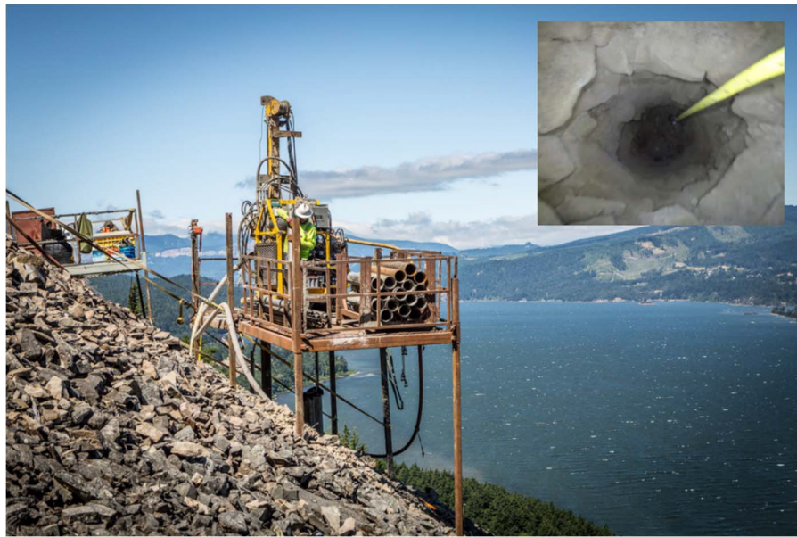
Figure 4. Drilling operations and downhole camera image (inset)
