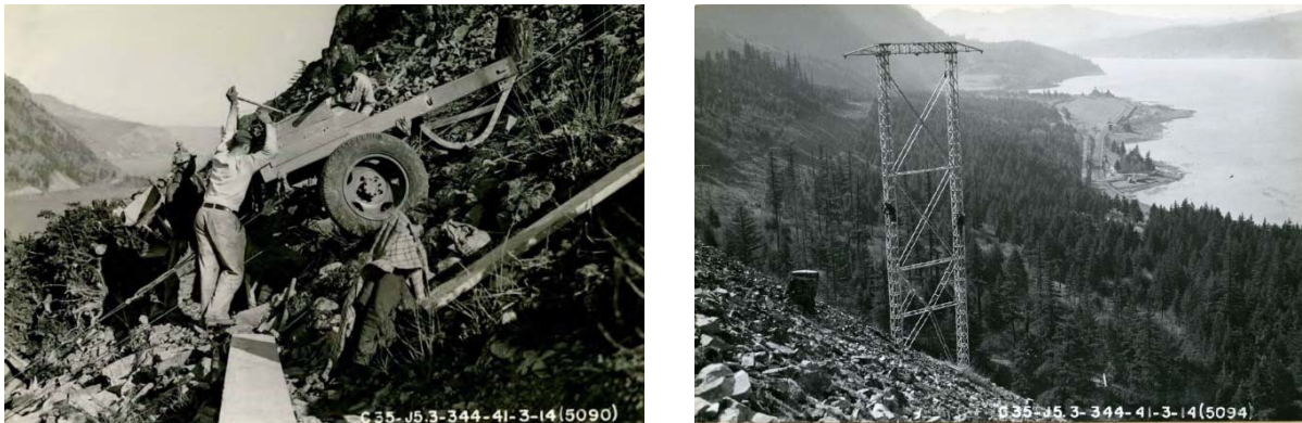
Figure 1. Concrete buggy pulled uphill via a winch and cable mechanism to hand place masonry backfill (left) and erected H-Frame tower (right)
